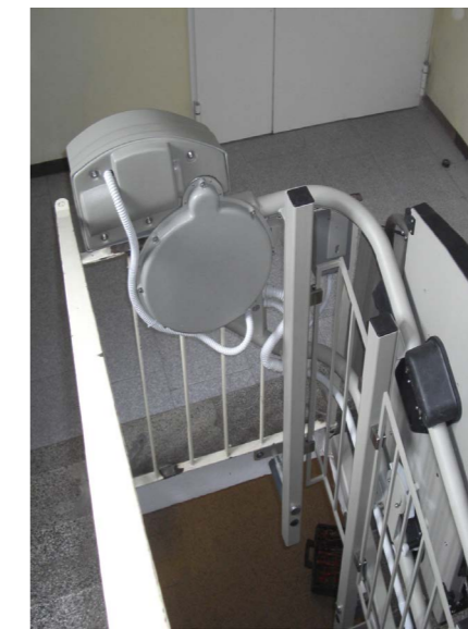
90° drive in the eye of the stair.
