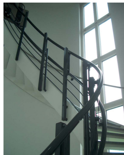
Fixing on the stringer
